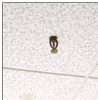
▲ Sprinkler head and smoke detector with Fine Fissured ceiling
