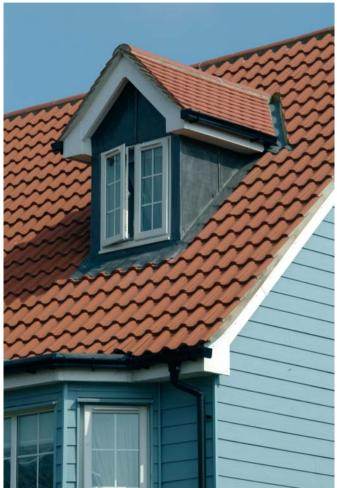
A single-lap interlocking concrete tile with the classic clay pantile profile.
