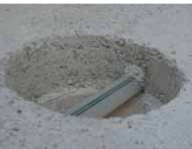
A heating pipe in the glaster® screed
