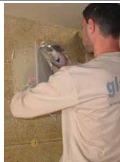
Internal glaster® plaster being applied to Tŷ-Mawr wood wool boards.
