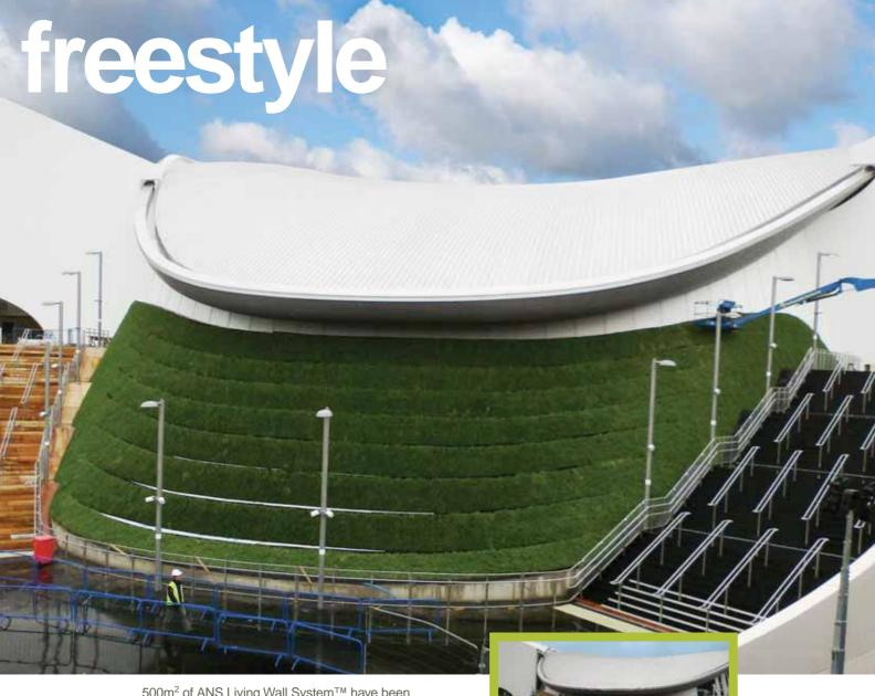
500m² of ANS Living Wall System™ have been supplied and were installed on the Aquatic Centre. After extensive research by the architects involved in the project, the ANS Living Wall System™ was the only system that could handle the complex curves and angles of the structure.
