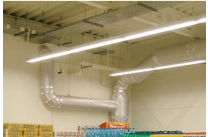
Connecting the ground-air heat exchanger and ventilation control centre
