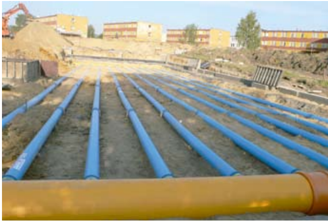
Ground-air heat exchanger using the Tichelmann system
